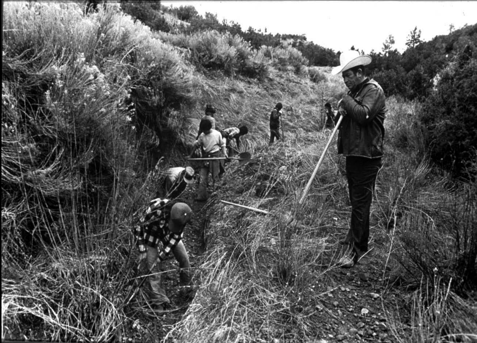
Ditch Cleaning at El Valle 1980
